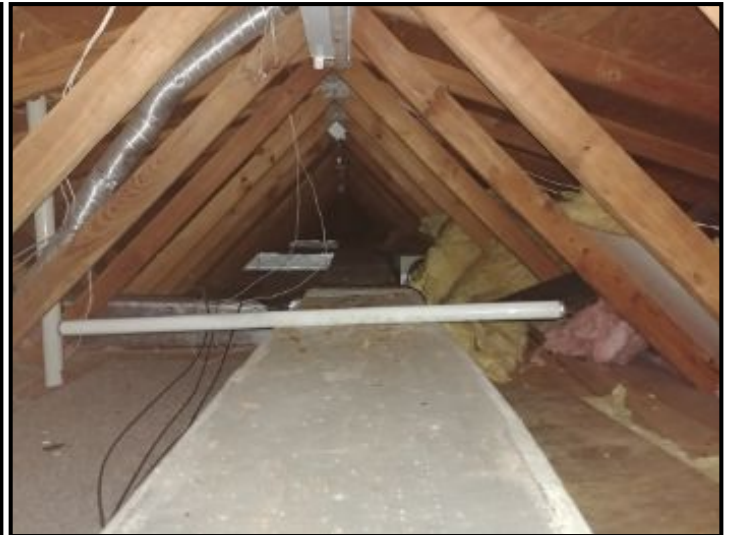
Attic rafters and venting
