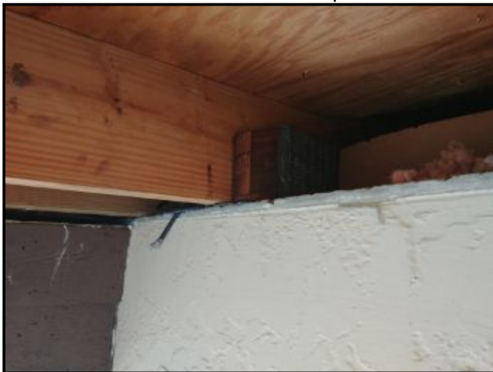
Rear roof connection at block wall/patio
