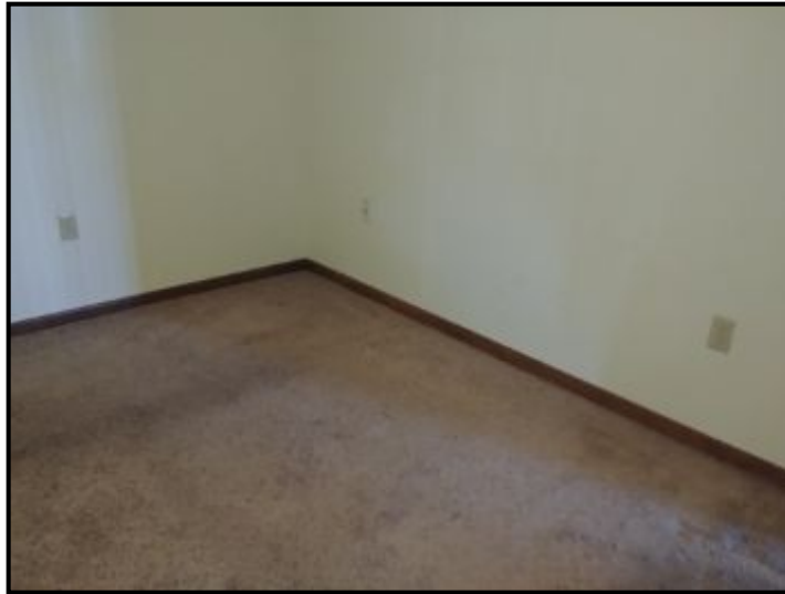
No AFCI breakers in BR
