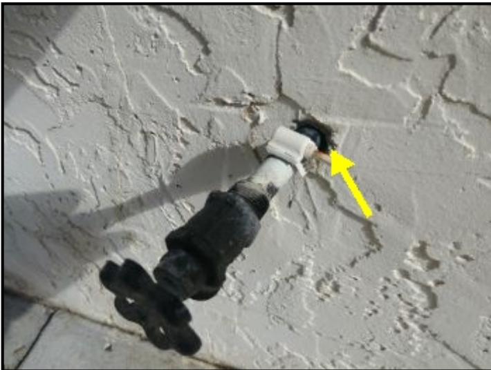
Pipe not sealed into house
