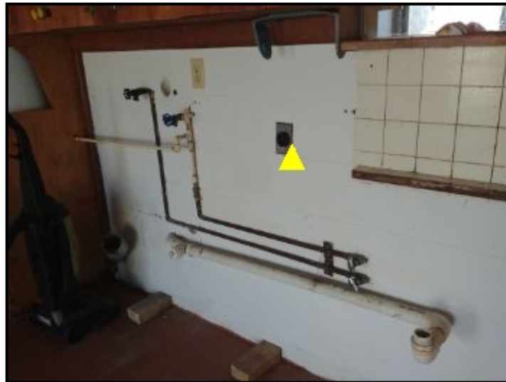
Laundry/sink connections and basin sink drain w/ 240 outlet
