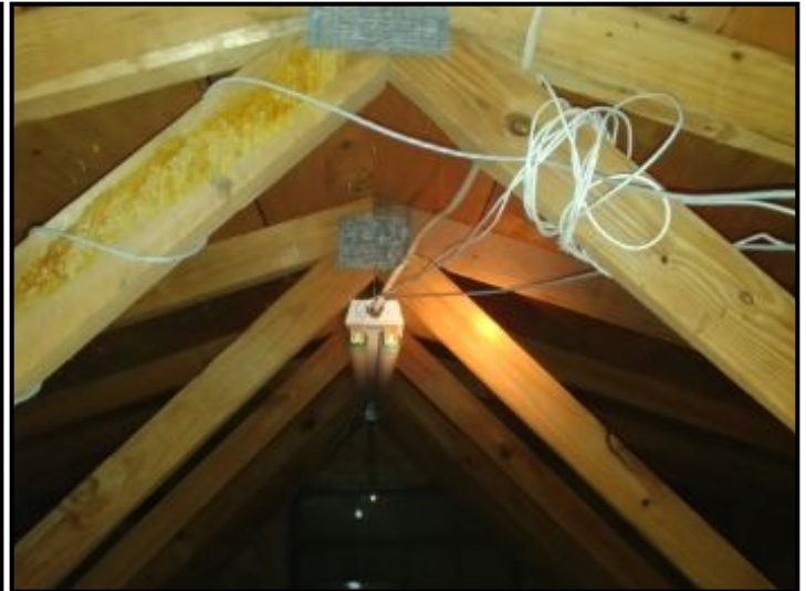
Unsecured wires
