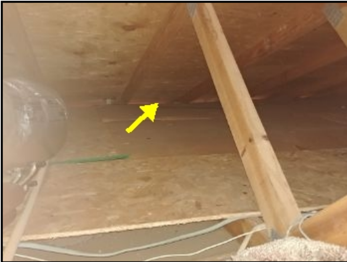
Attic space to soffit vents
