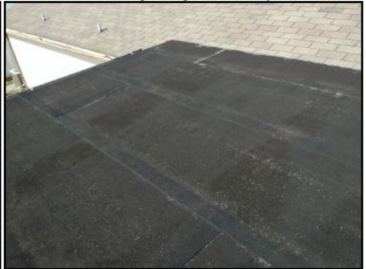
Roll roofing on rear patio
