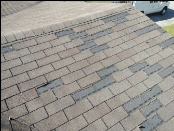
Broken shingles
