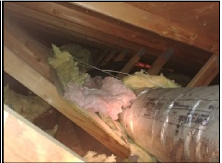
Attic insulation/AC duct
