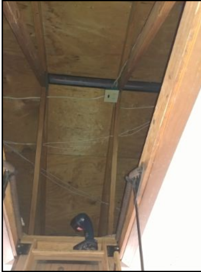
Pull down ladder in garage
