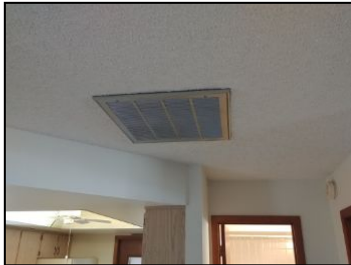
AC return LR ceiling
