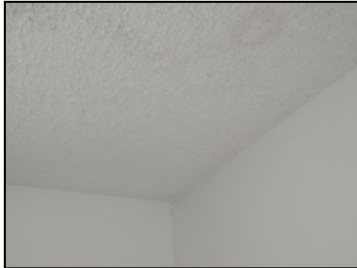
Interior Areas Ceiling Condition
