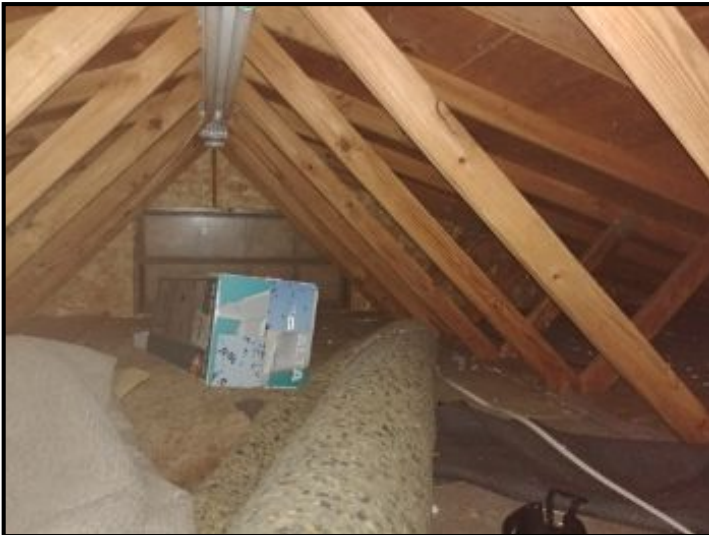
Rafters over garage area
