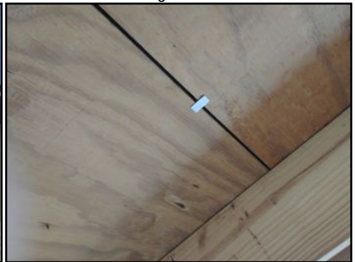
H clips present on plywood sheathing 1/2 in
