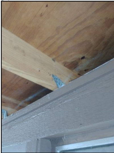
Rafter connection at back patio wall
