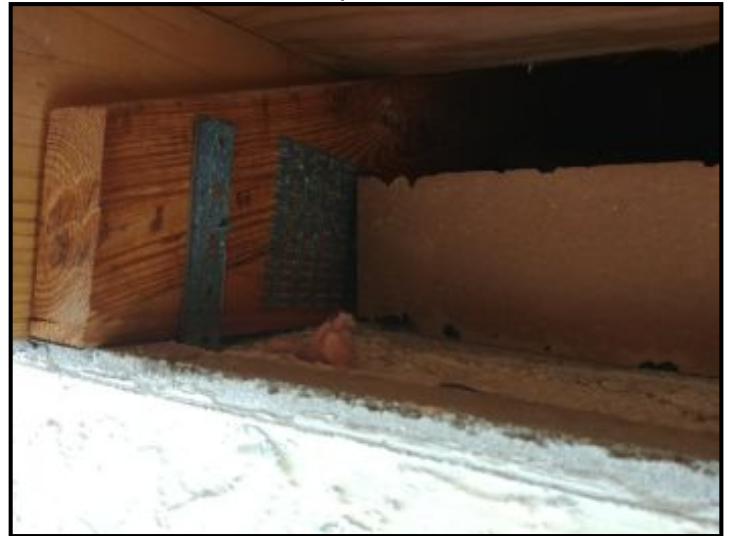
Connections to block and rafters
